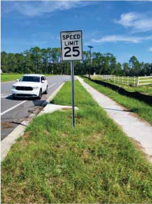
**Location 6:** Speed limit sign leaning and not 7' from the ground to the bottom of the stop sign.
