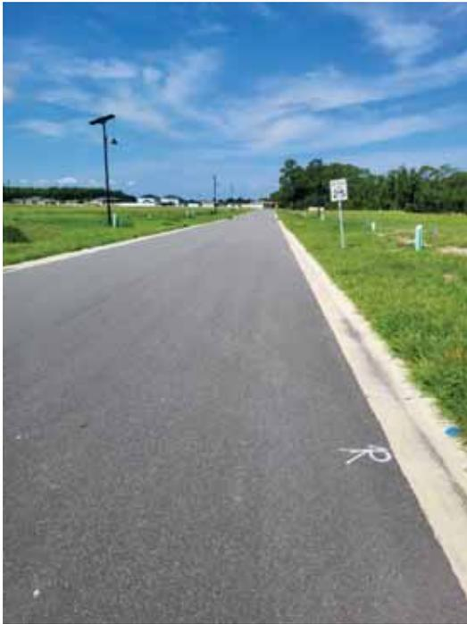
**Location 11:** Stop Sign leaning and not 7' from the ground to the bottom of the stop sign.
