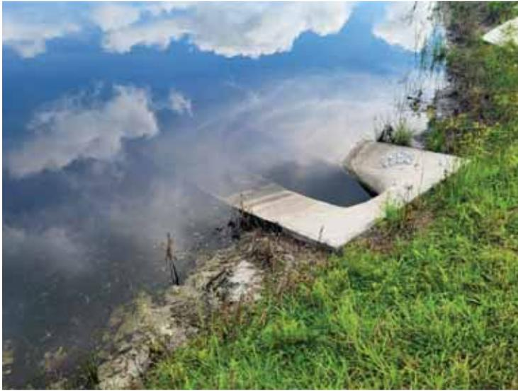
**Location 4:** Mitered End Section starting to erosion around the sides.
